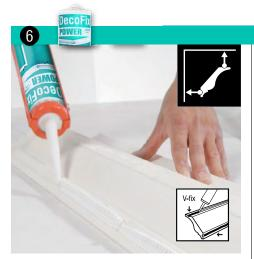
Apply DecoFix Power in V-Fix over the entire length | To apply an adequate quantity of Decofix Power, first take a stanley knife and trim the nozzle at 45deg allowing an appliction of at least 8mm diameter of adhesive. Use the V groove on the back of most cornice mouldings to guide the nozzle as you apply adhesive. Note the V groove of the coving will not stick to the ceiling if adhesive is only hidden within the V groove, the adhesive must overspill the indentation to work.
