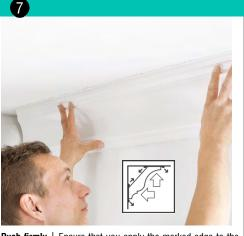
**Push firmly** I Ensure that you apply the marked edge to the ceiling. Put the coving into place, checking that it is horizontal and symmetrical to the wall and ceiling. When you are confident the coving is positioned correctly, firmly press it to the wall and ceiling across the entire length.
