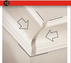
**Push** both mouldings firmly and securely together. Excess adhesive should seap through the joint.
