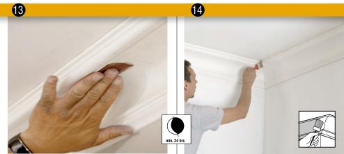
Prepare for paint | All Orac Decor® mouldings already have a white primer applied, but still need to be overpainted with a suitable paint. For good adhesion, lightly rub the length of the moldings with a 320 gram sandpaper.
