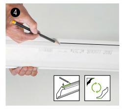
Marking the ceiling side | Add a black line to the ceiling side of the coving. When cutting place black line edge at bottom of mitre box! With other words, flip the moulding.
