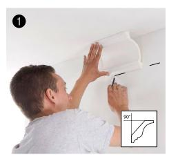
**Mark out** | Mark the bottom of the cornice on the wall. Make sure the moulding is positioned correctly at 90°
